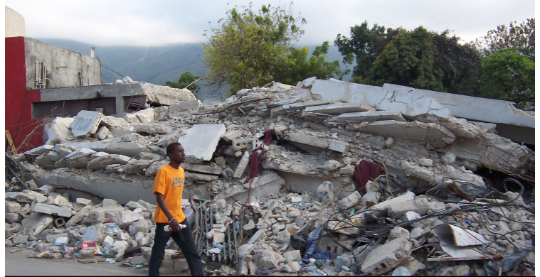
Rubble from the Earth Quake in Haiti
